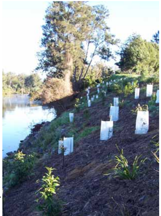
Lavenders Bridge, Bellingen Lomandra in foreground; mulch and tree guards.
